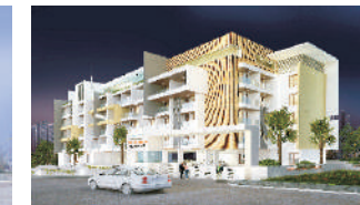
Shalimar Garden Old Kent Road, Mangaluru (Ongoing)
